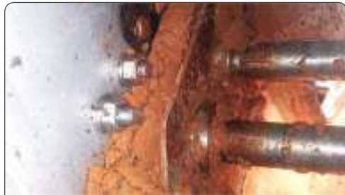
4 Dewatered Cake Outlet 脫水泥餅排出口
